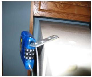
1. In this picture, a 2" x 1/2" x 1/8 " flat mending strip was screwed into existing screw hole on top of the refrigerator. These holes are also found in the space between the upper and lower compartments on the refrigerator. These holes are normally used to reverse the direction a refrigerator door opens. You simply remove the plastic cap that covers the hole and screw on the strip.
