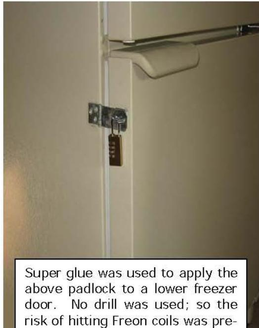
Super glue was used to apply the above padlock to a lower freezer door. No drill was used; so the risk of hitting Freon coils was prevented.
